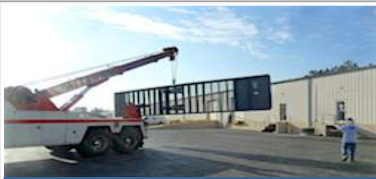
3. Wrecker pulls ramp right up to dock.
