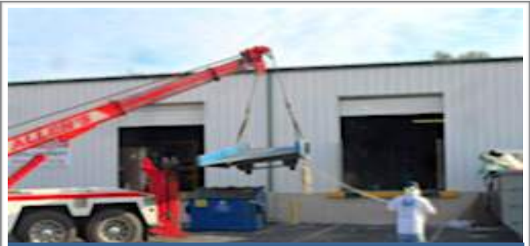
4. Wrecker takes ramp from flatbed to dock.
