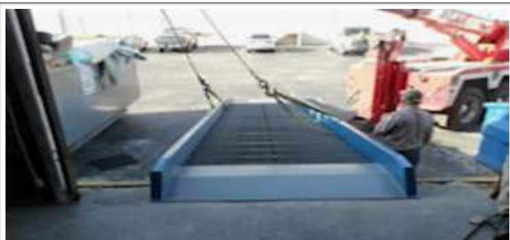
5. Ramp is in place.
